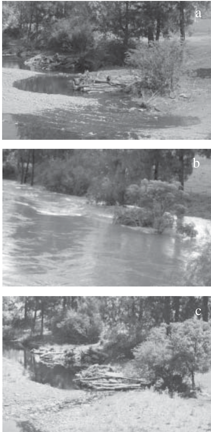
FIGURE 11. View from upstream of 2 of 15 engineered logjams constructed in the Williams River, northwest New South Wales, Australia. (a) As-built structures in September 2000, (b) March 2001 flood during which peak flow overtopped structures by approximately 2 m with velocities exceeding 3 m/s, and (c) same structures in 2002 after six overtopping flows.
