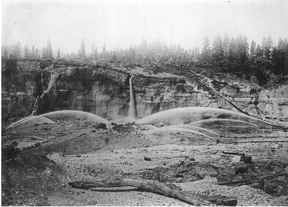
Fig. 9. Hydraulic mining at the Malakoff diggings of the North Bloomfield Gravel Mining Company in the Sierra Nevada (Plate A from Whitney, 1880).
